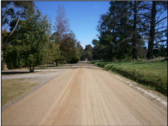
Figure 5: Allan Street - View West
