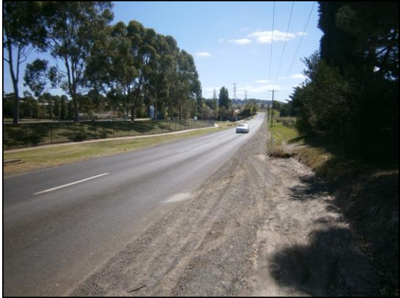
Figure 3: Manuka Road - View North
