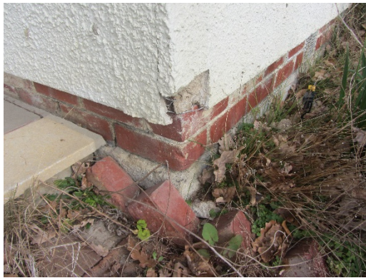
Figure 7. Concrete strip with two courses of red brick for providing base wall (Source: Context 2017)
