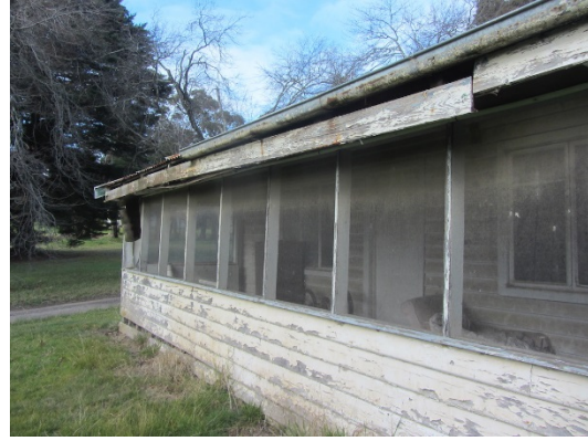
Figure 5. Detail of verandah showing fly screen enclosure (Source: Context 2017).
