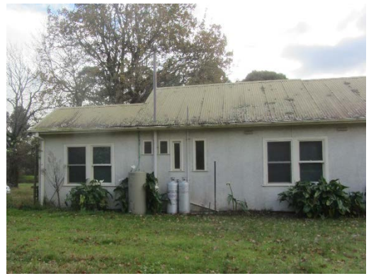
Figure 10. South view with original timber windows (Source: Context 2017)
