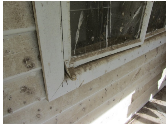
Figure 9. Detail of steel casement window (Source: Context 2017)
