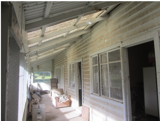
Figure 8. View of verandah leading to bedrooms (Source: Context 2017)
