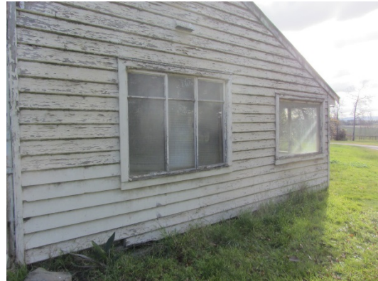
Figure 7. East view of bedroom wing (Source: Context 2017)
