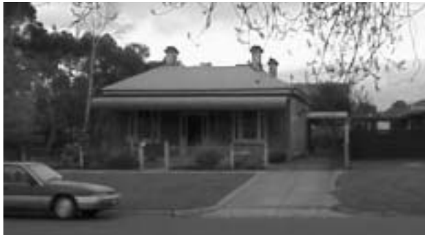
St. John's Vicarage, Bakewell Street Cranbourne. Built 1889
